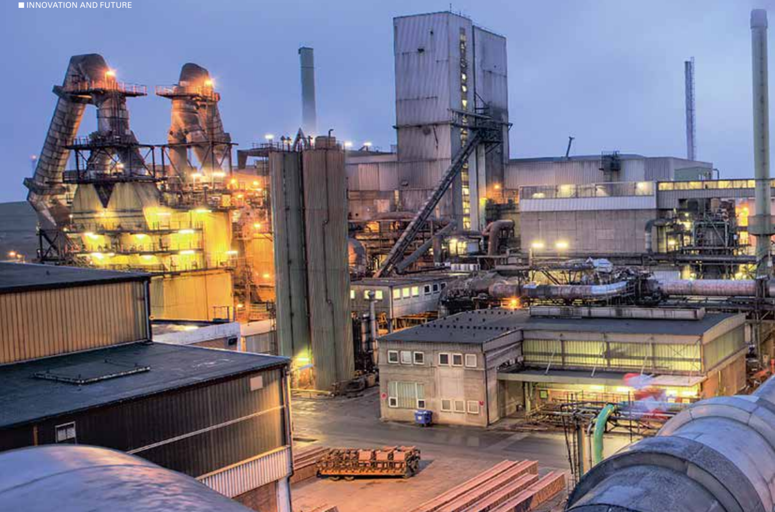
Aurubis derives heat from what is known as the contact acid plant, in which the gaseous sulphuric oxide formed in the process is converted into liquid sulphuric acid. The plant consists of three lines. Around 160 million kilowatt hours (kWh) of heat per year can be derived from each of these.
