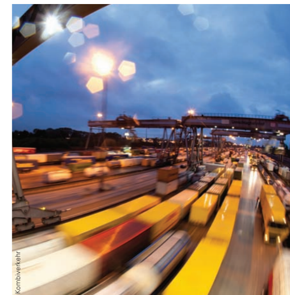
The Billwerder Terminal handles continental intermodal services.
